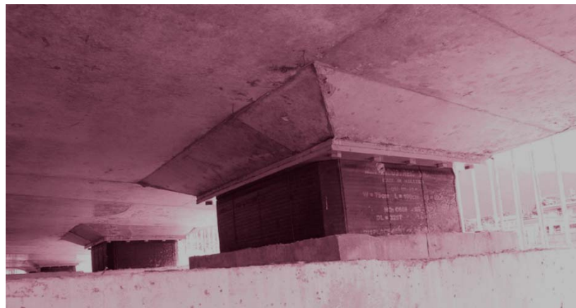
Figure 21 Photo of Lead Rubber Bearing
