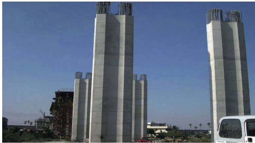
Figure 24 Photo of pier using self-compact concrete, smooth surface
